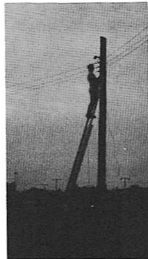
W3LHF "BORROWING" POWER K3MXM HOLDS THE LADDER
